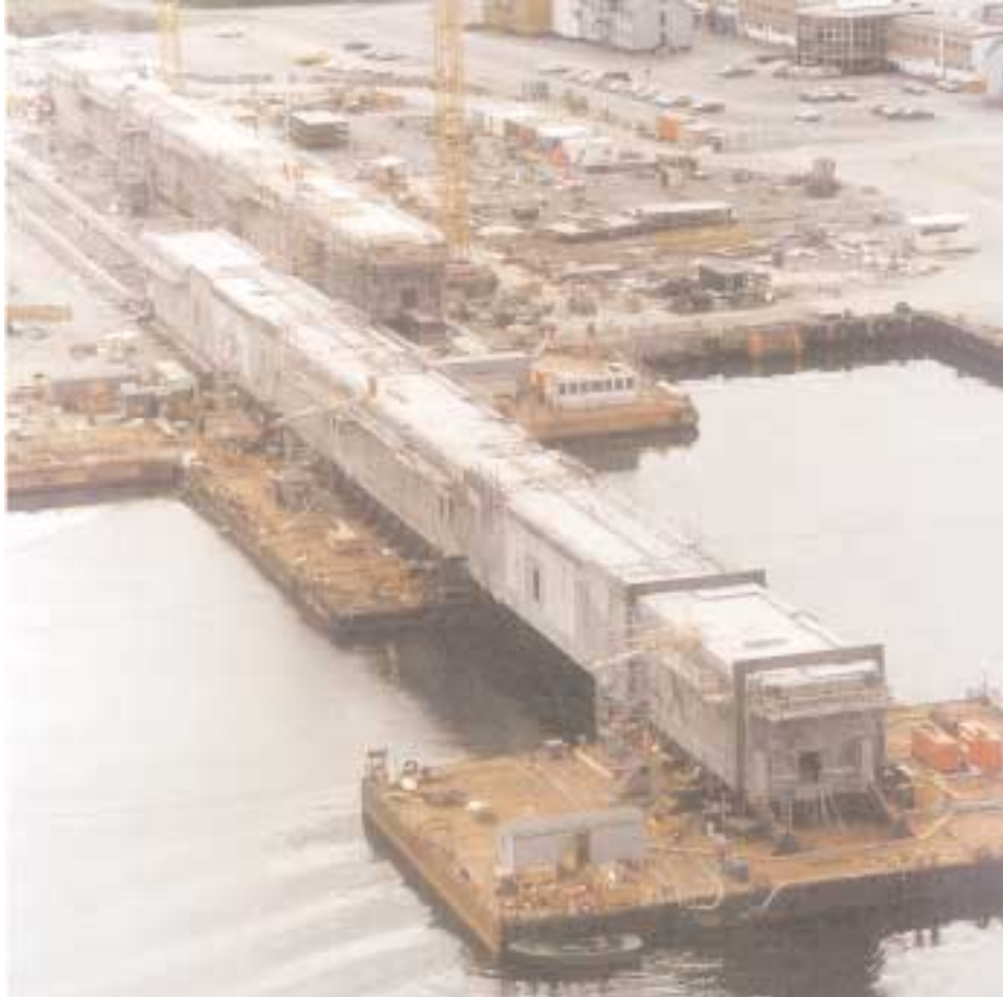
The first module support beam during launching
