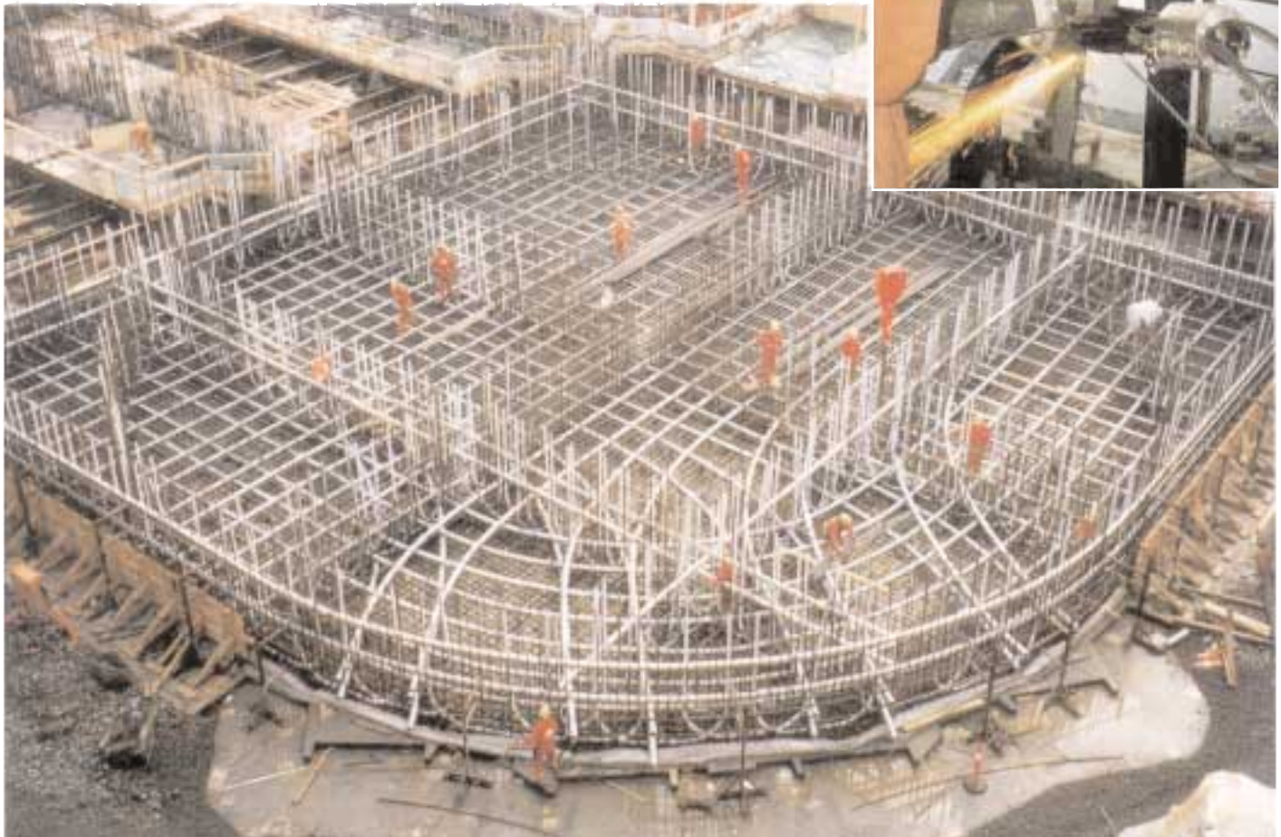
Duct placing in bottom slab
