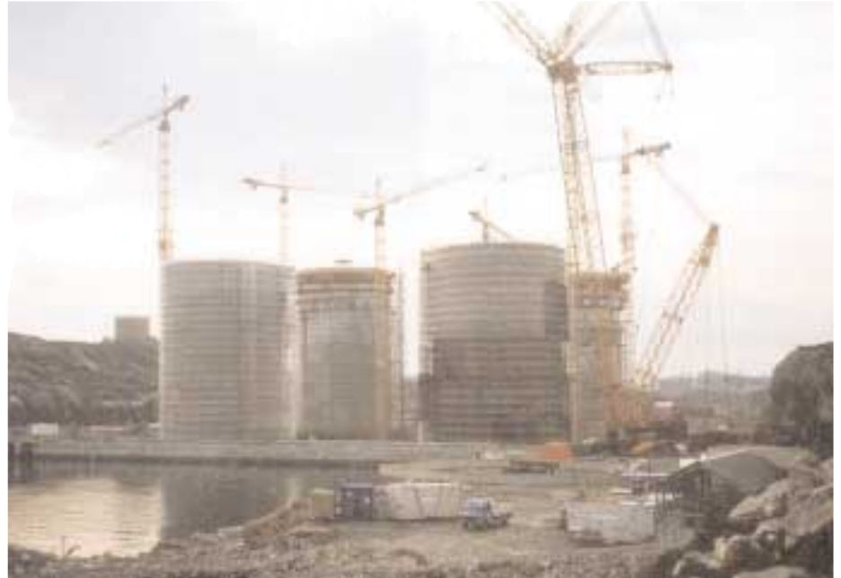
Slipforming of the columns almost complete
