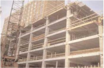
16 inch x 28 inch beams span 52 feet. The slabs employ VSL SA anchorages with 1" x 3" PT-PLUS plastic duct, encapsulating up to 4 strands. The typical beam employs one EC 5-12 tendon. This represents a 42 % reduction of end bearing area, when compared to individual monostrand anchorages. The use of the bonded components reduced congestion (when compared to the unbonded system) and helped the contractor achieve an aggressive construction schedule.
