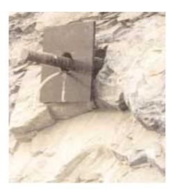
Electrically isolated passive bar anchor
