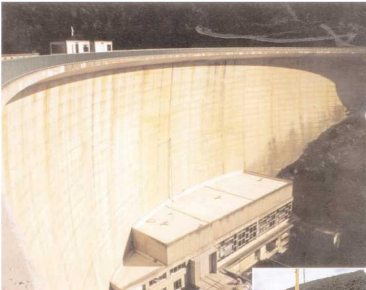
To increase the overall stability of the Esch sur Sure dam, located in the northern part of the Grand Dutchy of Luxembourg, the utilisation of permanent rock anchors was proposed.
